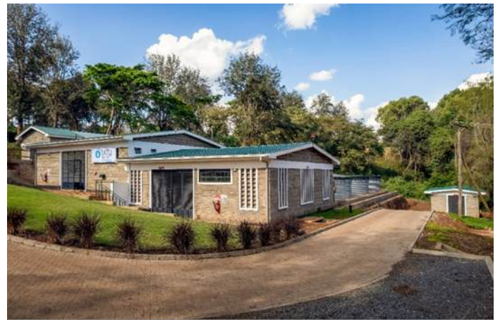
Figure 23: Water Treatment Plant 2026
