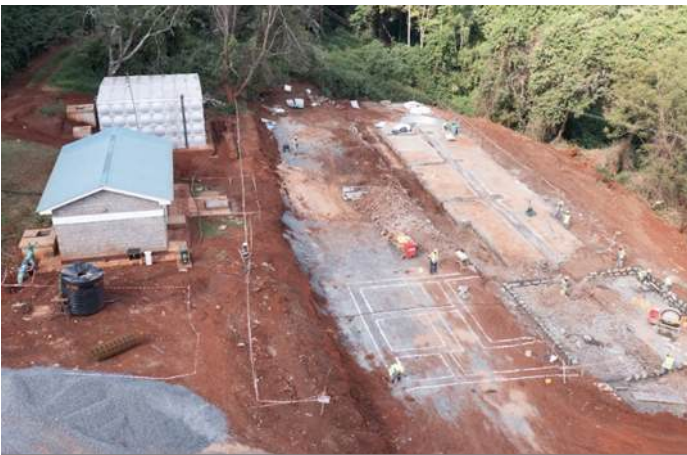
Figure 22: Water Treatment Plant 2022
