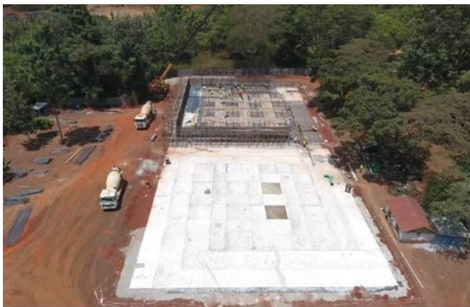
Figure 24: Water storage tank site 2022
