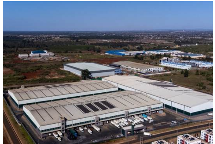
Figure 19: Tatu City Industrial Park 2026
