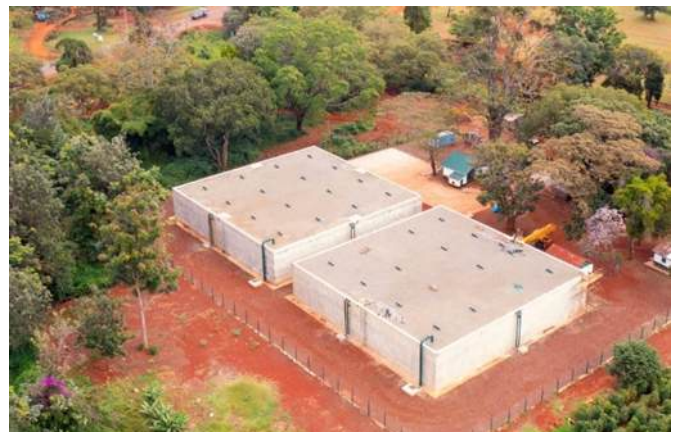
Figure 25: Water storage tank site 2026
